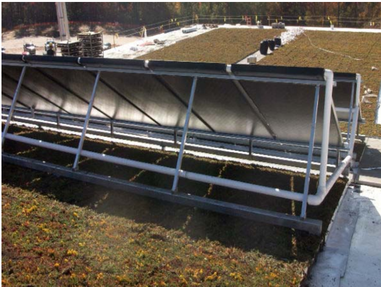
Green roof on park facility
