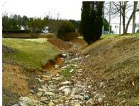
Receiving Channel - Before
